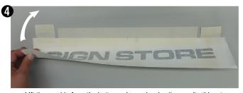
Lift the graphic from the bottom edge and swing it up on its "hinge".
