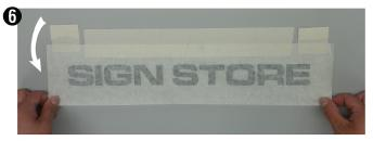
Hold the transfer tape by the two loose corners and swing the graphic down on the "hinge" until it comes in contact with the application surface. Press the corners down to hold the graphic in place.
